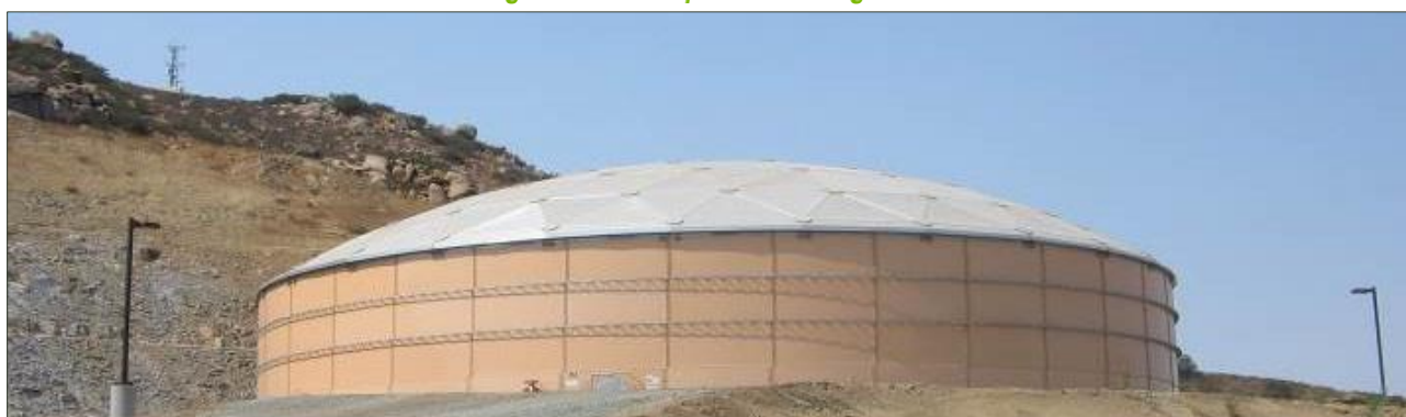
Figure 29: Example of a storage tank
